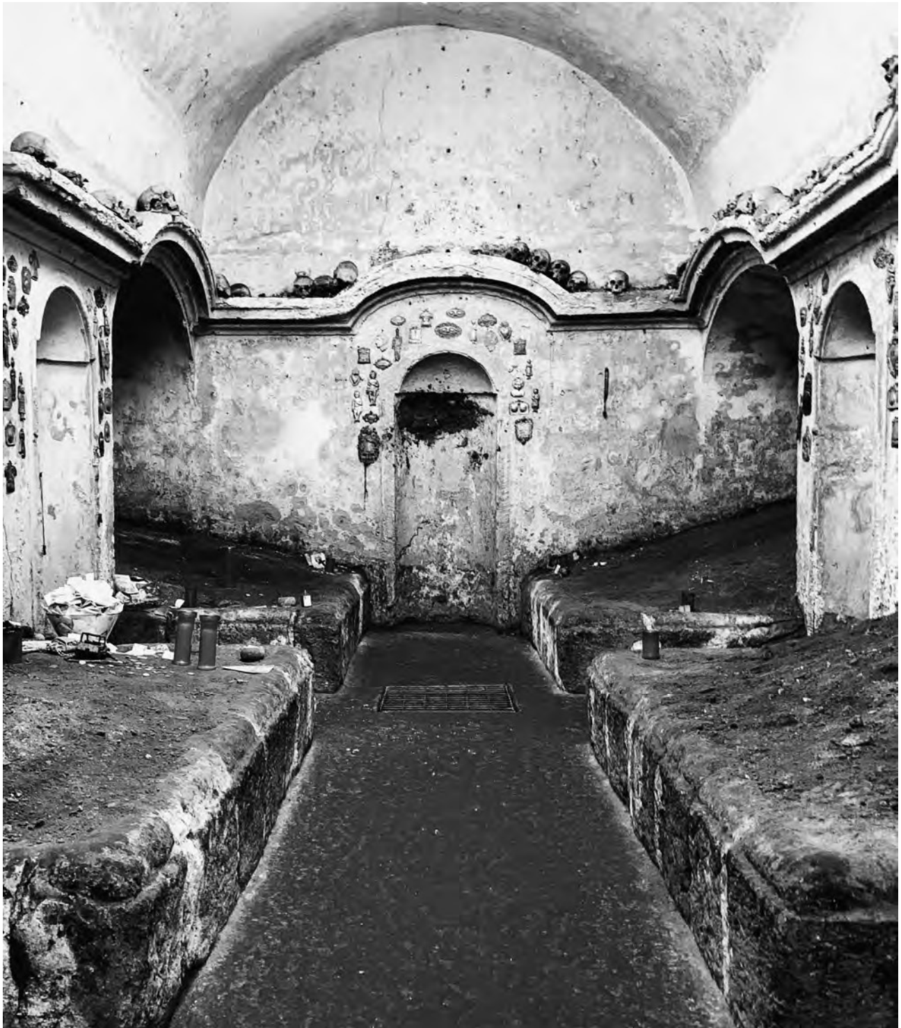
FIGURE 1: Typical structural organization of a terrasanta: a vaulted room with four "giardinetti", a central corridor and niches; above the latter a ledge for the laying of the skulls runs along the walls; in the middle of the corridor one can see the grate that gives access to the ossuary below. (Church of Santa Luciella, Napoli.)
