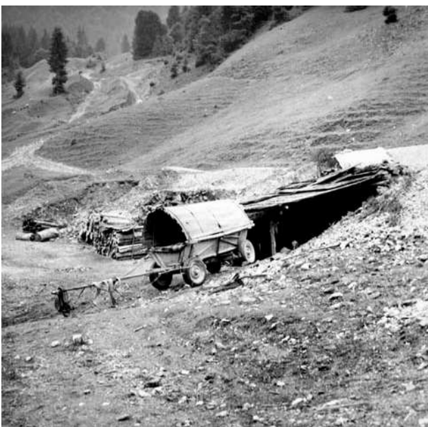
FIGURE 7: Maramures, Rodna, traditional sunken lime pit before the selection of burnt lime. Photo by Jan Jelínek 7/10/1974.
